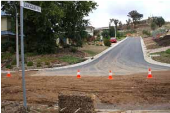
Figure 4: Debris flow deposit in Chapman, Canberra February 2007. The mud and hay bale were transported down the street by fast flowing water during a heavy downpour.
