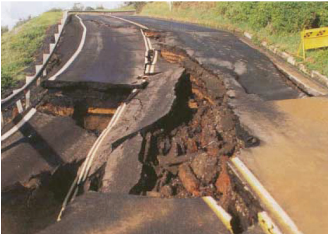
Figure 8: Debris slump on Lawrence Hargrave Drive (UoW website, photo: Flentje)
