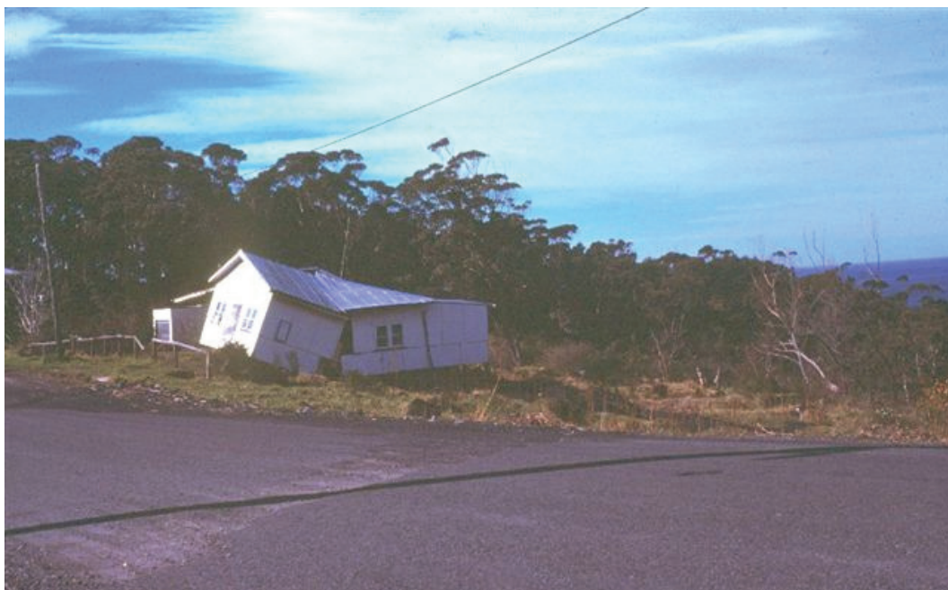
Figure 16: Major structural damage to house on Morrison Avenue during 1974. Damage resulted from house straddling landslide margin. Photo by Ann Young, accessed from UoW website on 20 January 2009.
