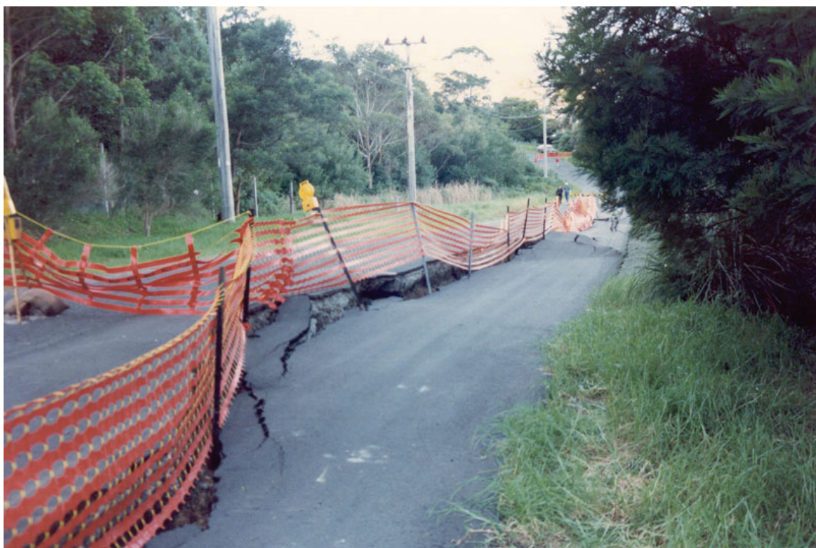
Figure 14: Damage to the pavement of Morrison Ave, in April 1990. Photo taken by Phil Flentje and accessed from UoW website on 20 January 2009.
