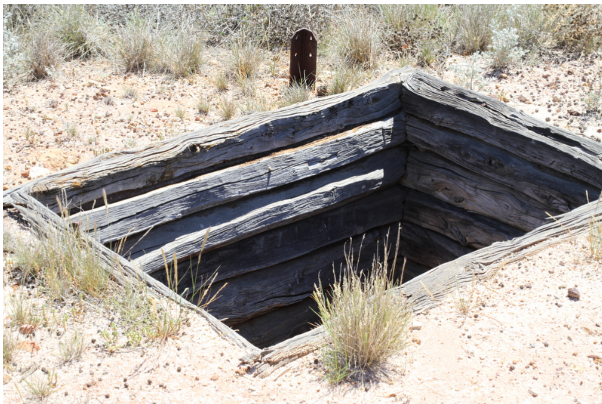
Figure 40: A hand-dug well lined with timber in the Kingoonya Palaeovalley area (photo by Evgeniy Bastrakov, November 2010).
