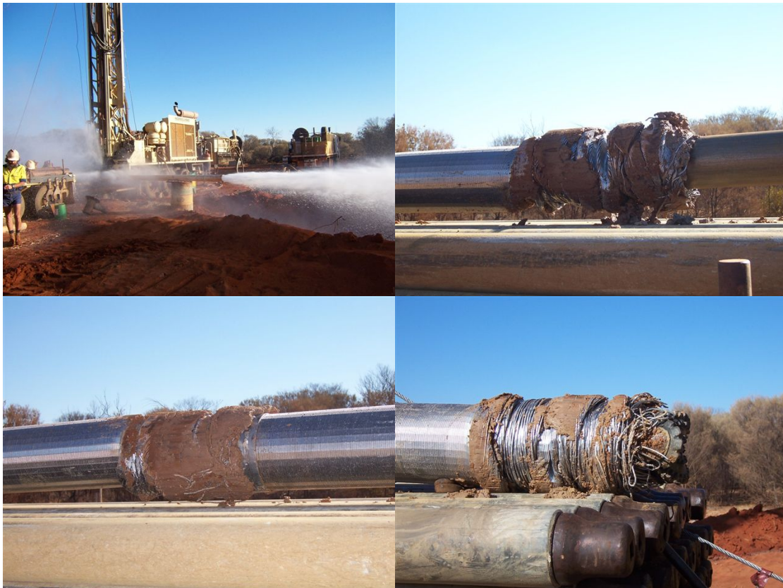
Figure 4.8: Drilling operations at RN 18356 highlighting the damage caused to the in-line screens due to problems in constructing the borehole.
