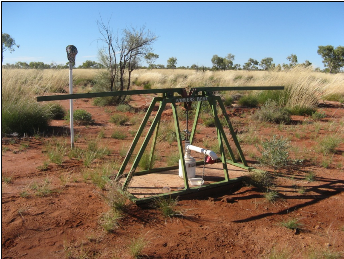
Figure 3.20: The handpump mechanism installed at Winner's Bore on the Nyirripi to Kintore road as an emergency water supply.
