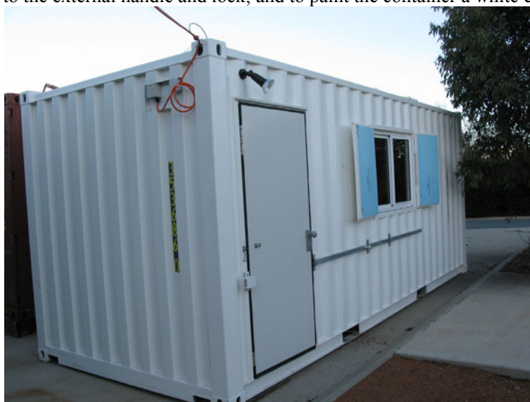
Figure 8: Container after modifications including installation of double glazed windows; spotlight, security bar and insulated metal shutters
