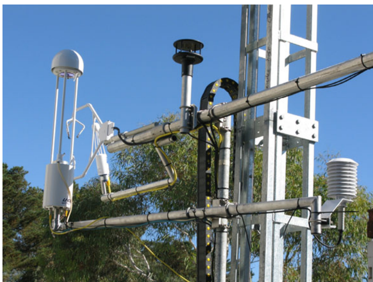
Figure 17: EC equipment and tower tested at Geoscience Australia before deployment
