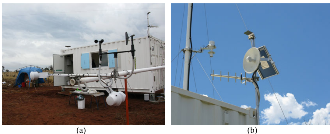
Figure 5: a) Temperature and relative humidity sensors mounted in a Gill radiation shield on cross arm (left) and RM Young Wind sentry set (right) (mast in lowered position); b) solar panel for weather station, top mounted pyranometer, dish for wireless connection to EC tower and Yagi Antenna for internet communication
