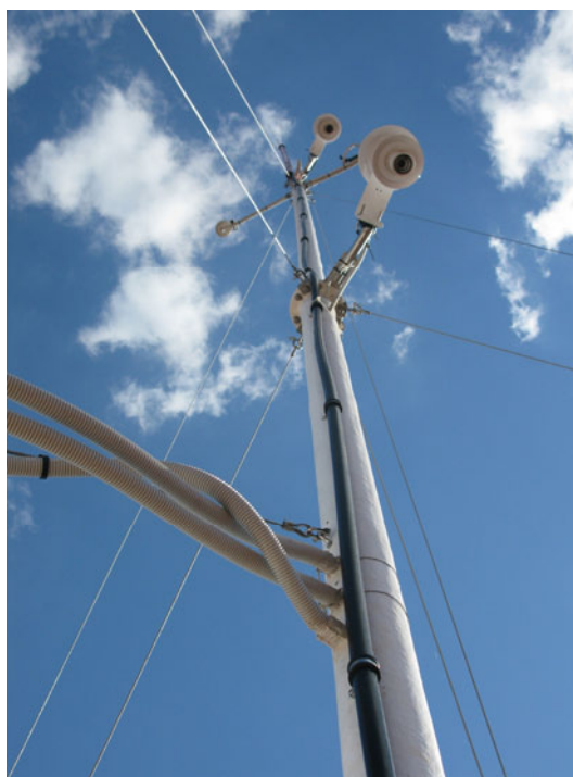
Figure 3: Mast and air intakes at 5m and 10m height.
