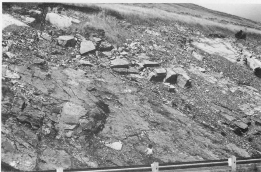
Fig. 7. Slab slide in road cutting south of Adelaide.
