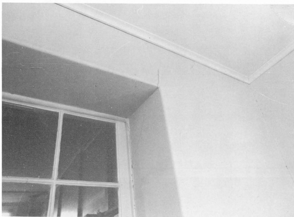
Fig. 3. East-west internal wall, cracking over window and at corner.
