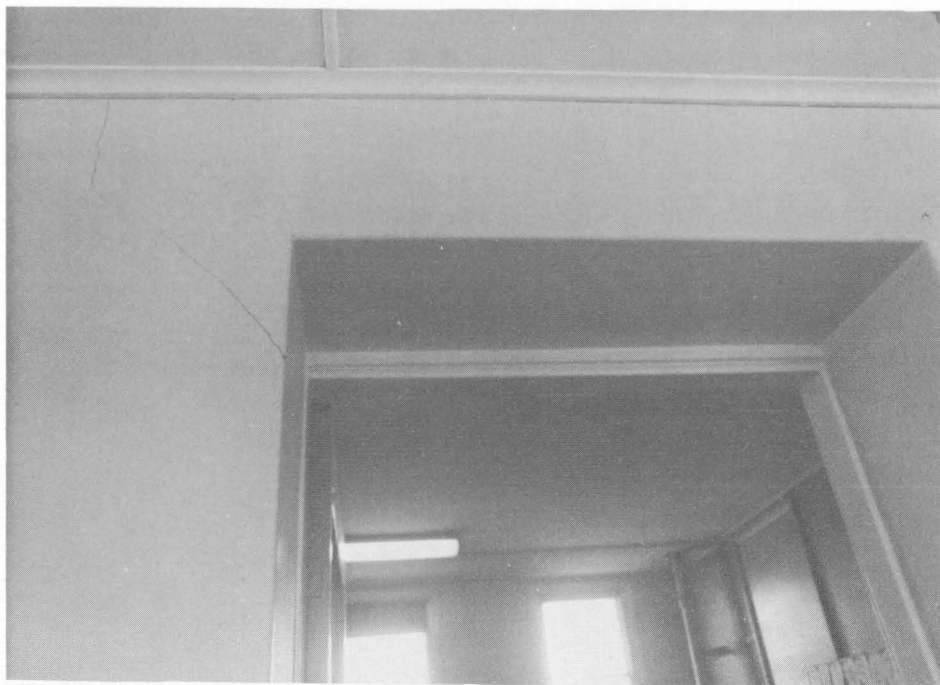
Fig. 2. East-west internal wall, 2-mm-wide crack at doorway.
