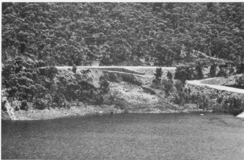
Fig. 6. Recent landslide on edge of Kangaroo Creek Reservoir.
