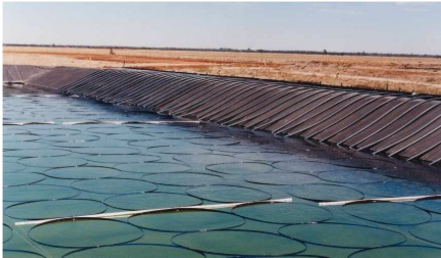
Figure 1.7 A solar pond at Pyramid Hill (near Kerang in Northern Victoria) showing the mesh of pipes running down the wall of the pond. These run across the bottom of the pond and up the other side. Fresh water (or radiator coolant) is circulated through them, and is heated by the saline pond water. This hot fluid is then used to heat air to flash dry gourmet salt products. The plastic rings visible on the surface of the water are used to reduce water movement caused by wind ( http://soilwater.com.au/solarponds/ ).
