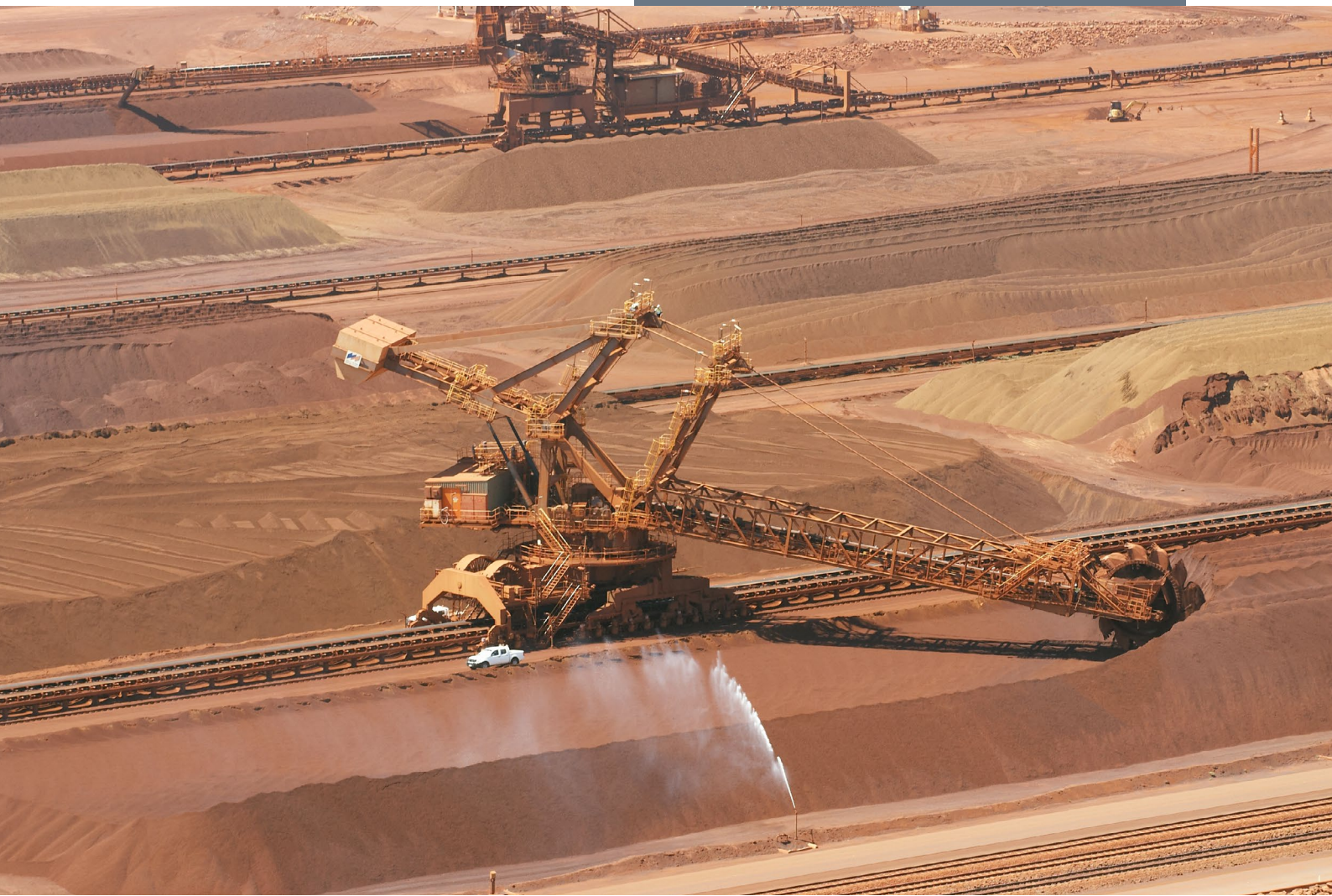
Photo: Aerial view of reclaimer working iron ore stockpile at Karratha shipping terminals, Western Australia.
