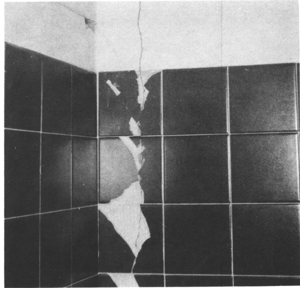
Figure 6. The vertical crack in Figure 5 continues down into the tiles in the lower part of the wall.
