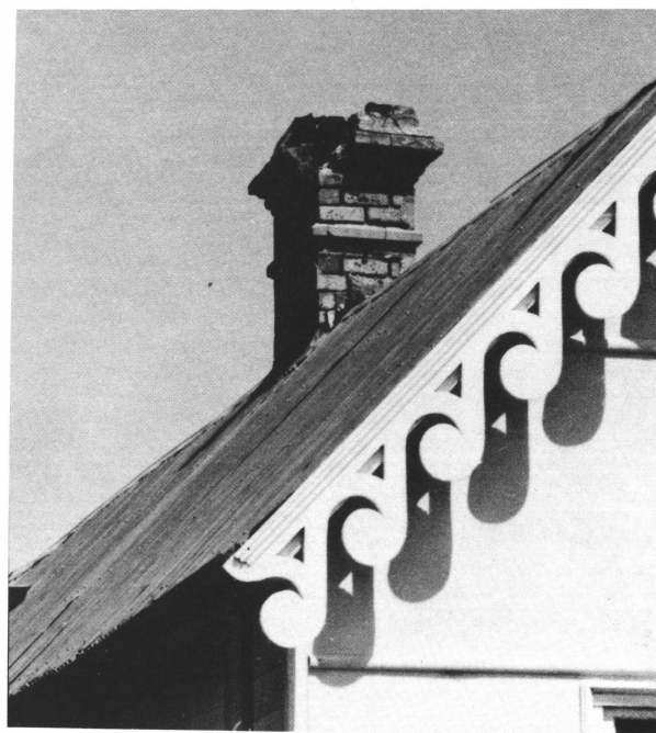
Figure 3. Earthquake-damaged chimney in Lithgow.
