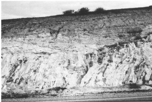
Figure 4. Road cut on Eyre Peninsula, South Australia, revealing underlying steeply dipping Precambrian rocks that have been weathered, differentially bleached and mottled. They are overlain by younger, horizontal palaeochannel deposits that have, in turn, been weathered and ferruginised in the top 2 m of the section. Note that the large mottles in the basal part of the section do not extend into the younger palaeochannel. Section is 7 m high.
