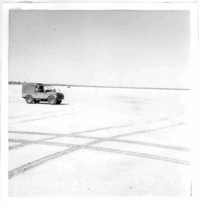
Lake Dora, showing the thin \frac{1}{8} " layer of salt on the surface, overlying 2 ft. of black mud containing Permian foraminifera. Once the surface is broken a vehicle will sink.
