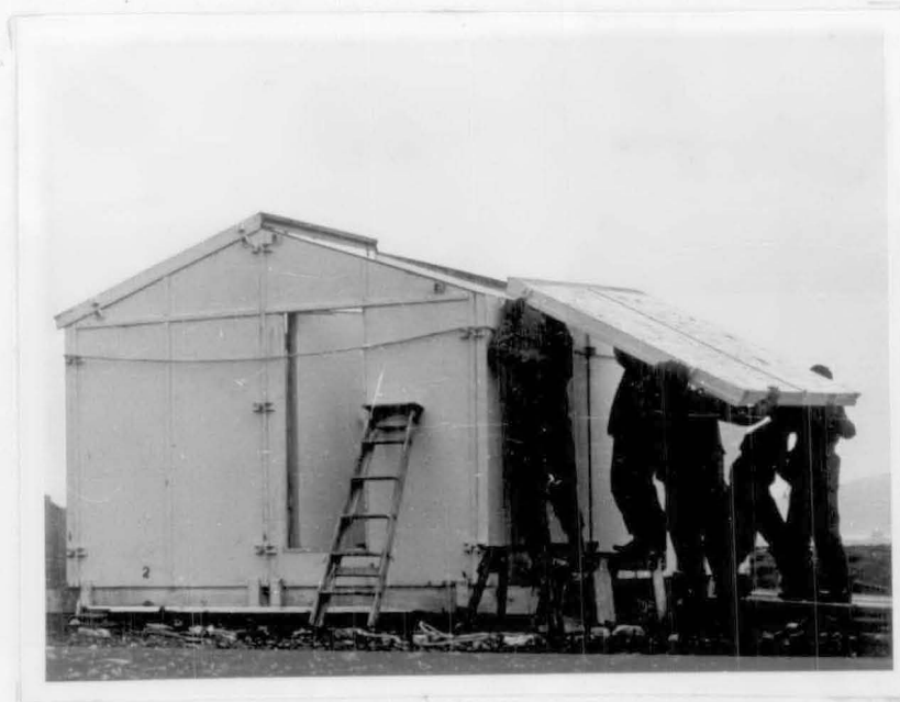
(a) Fitting the roof panel.
