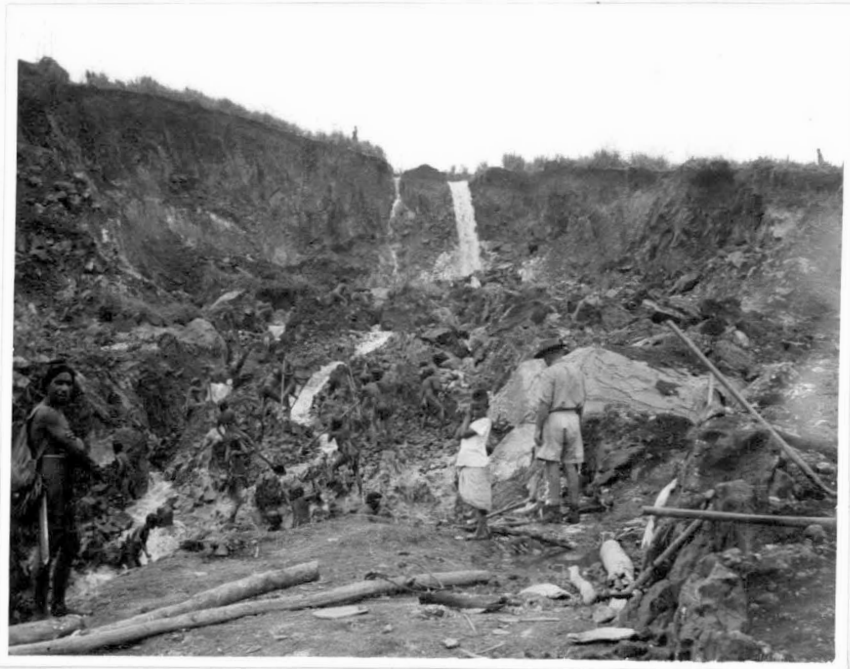
KUTA GROUND SLUICING EASTERN FACE OF NO.3 WORKINGS ON KUNIMO CREEK
