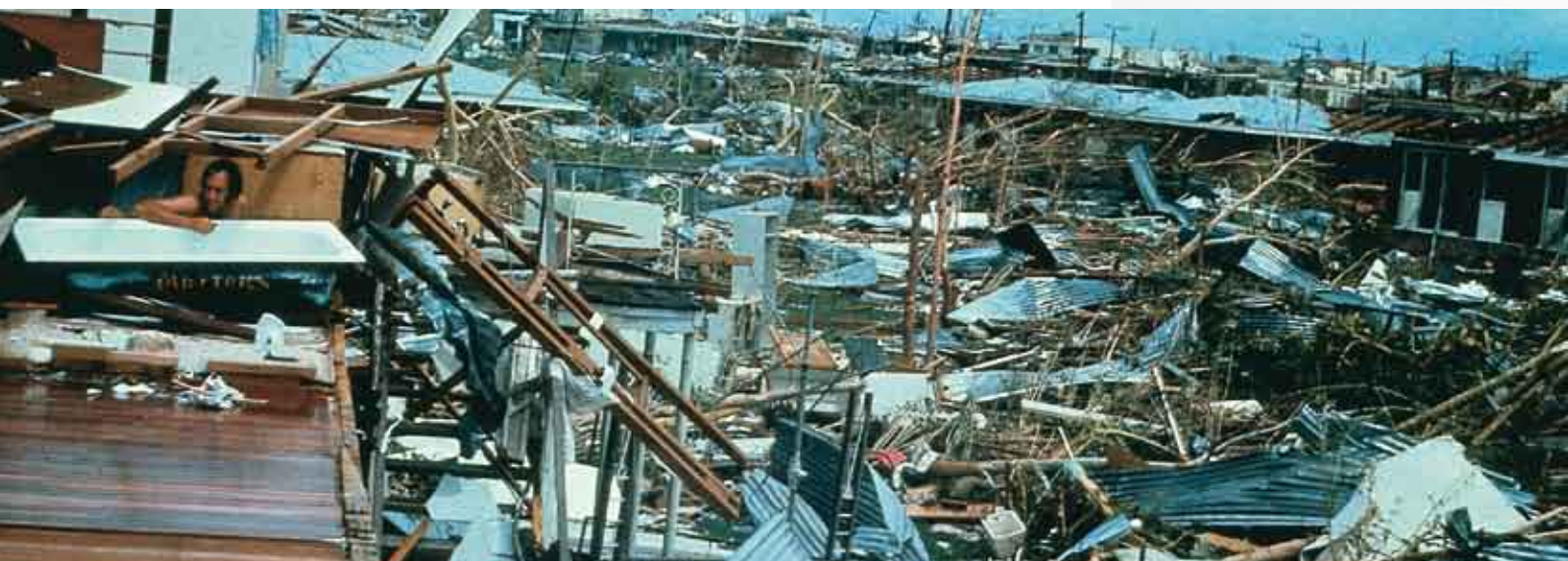
Damage to flats at Nightcliff from Cyclone Tracy in Darwin, Northern Territory, December 1974 Photo courtesy: Bureau of Meteorology/Noel Stair.
