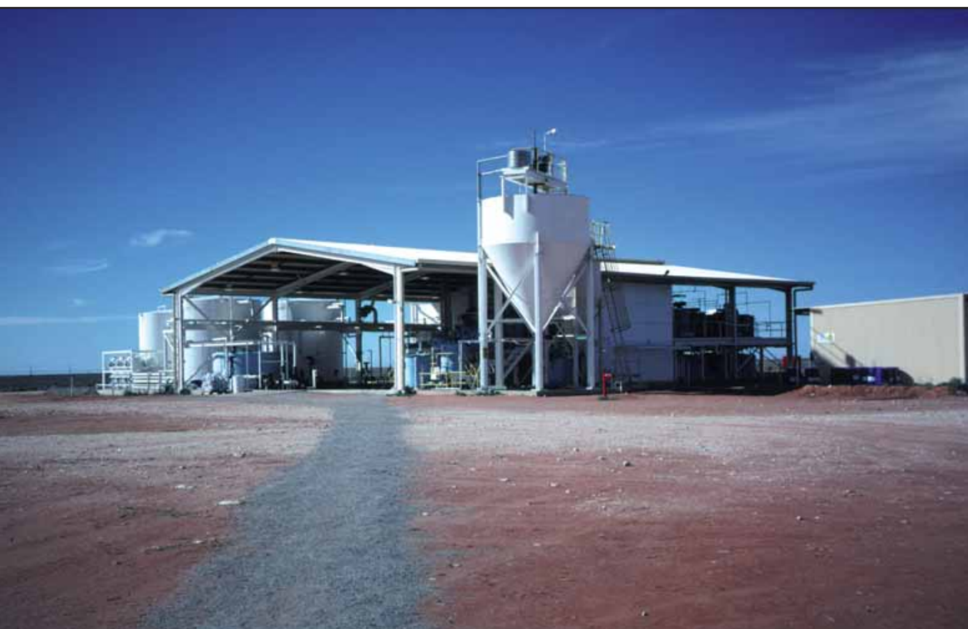
Plate 9 Solvent extraction demonstration plant at the Honeymoon uranium project, South Australia Photograph courtesy of Aden McKay, AGSO; published with the permission of Southern Cross Resources Australia Pty Ltd
