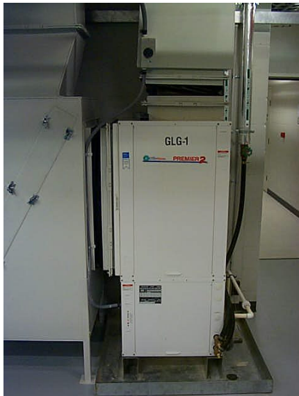
Fig.1: Typical Geothermal Unit
