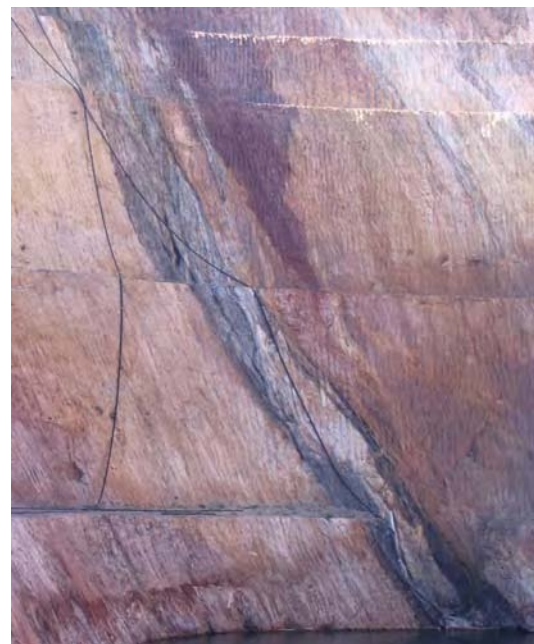
Steeply E-dipping shear in black 'shale' at centre of Parmelia pit
