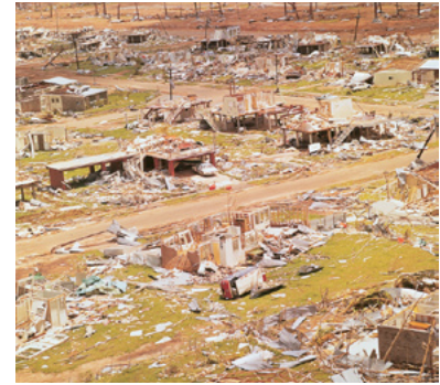
Figure 1. Destruction caused by tropical cyclone Tracy in Darwin, Northern Territory, December 1974. Photo courtesy of Bureau of Meteorology.
