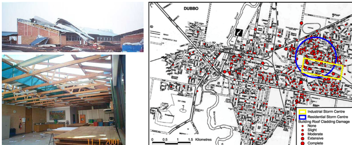
Figure 1. Wind damage - Yarrandale High school Photo courtesy of Mr Wilson - Site Foreman
