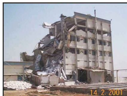
Figure 2. Damage from the January 2001 Gujarat earthquake
