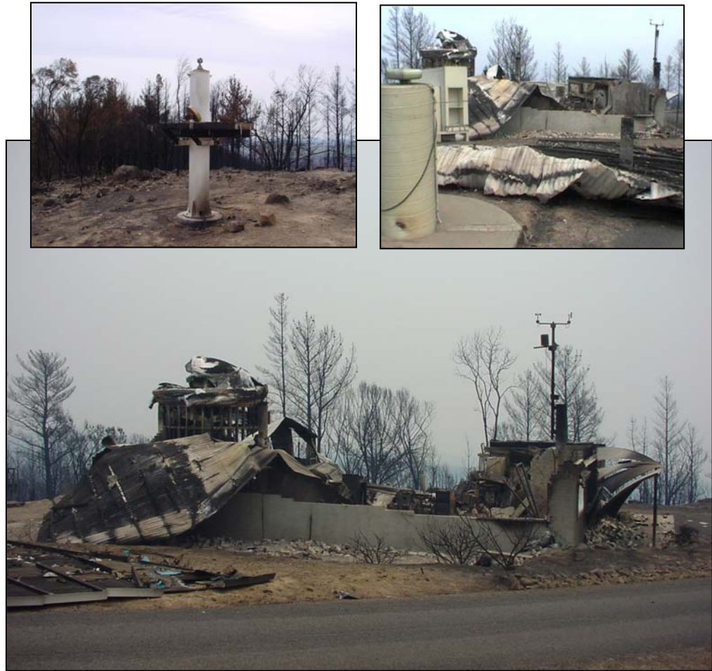
Figure 2: Mount Stromlo Satellite Laser Ranging (SLR) system. The Mount Stromlo fire damage. Bottom; Satellite Laser Ranging station post-fire. Top left; International GPS Service (IGS) station STR1 monument relatively un-damaged. Top right; Satellite Laser Ranging station post-fire with International GLONASS Service (IGLOS) station in the foreground.
