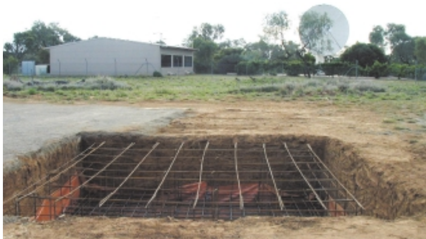
Groundwork for the additional X-Band antenna. Photo by Shaun Evans.
