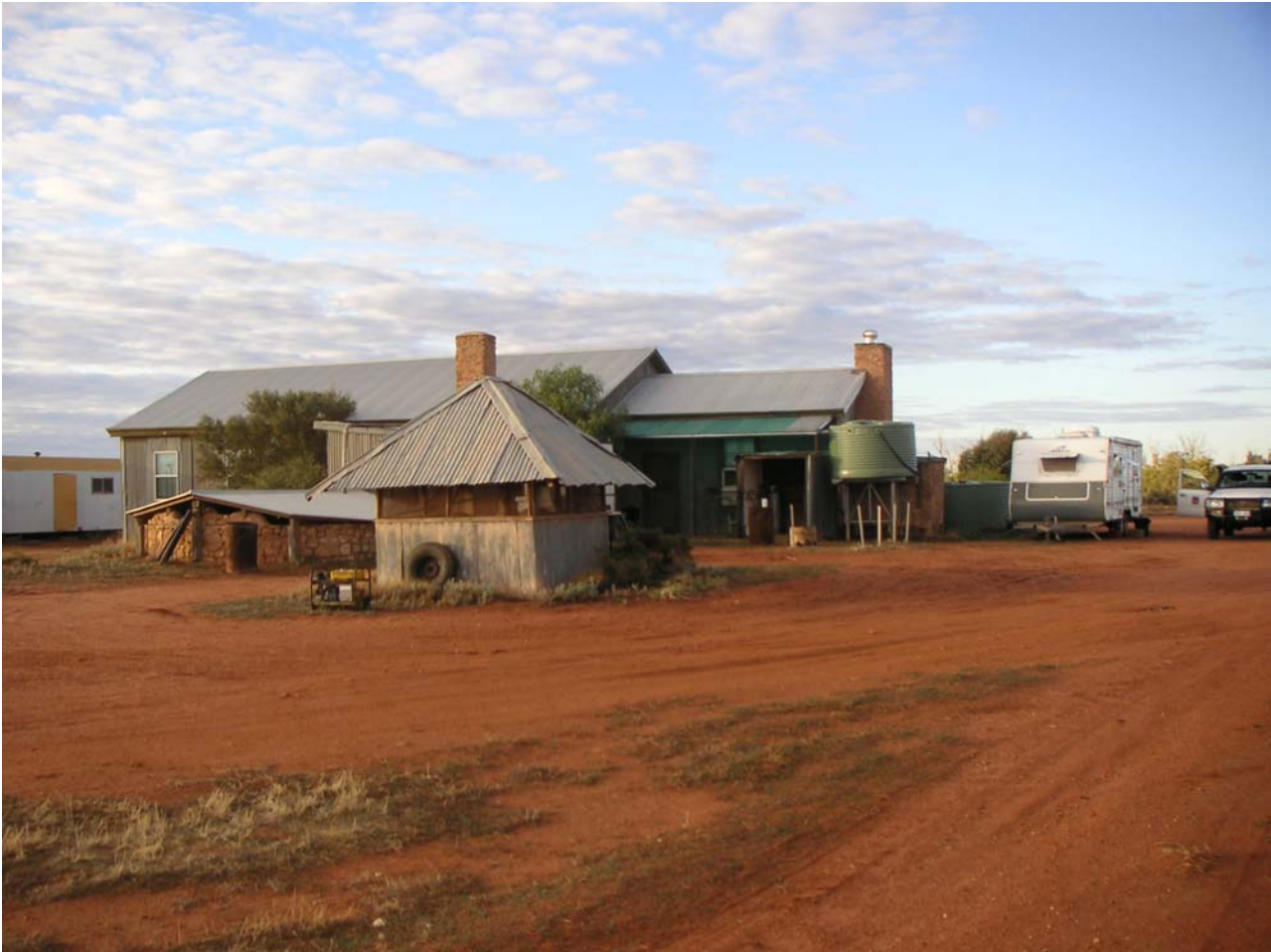
Figure 3. Accommodation at Curnamona station was in the shearers quarters.
