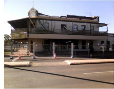
**Figure 2.** Damage caused to a hotel in Boulder. The damage is typical for two storey unreinforced masonry buildings with toppling of parapets either outwards into the street or inwards through the roof. This building also sustained other types of damage such as cracking over doors and windows and substantial cracking to internal masonry walls.
