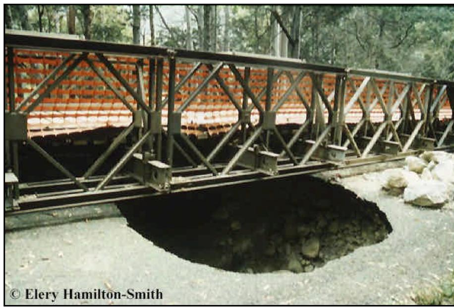
**Figure 1** Road collapse due to inappropriate location of road. (Photograph courtesy of Etery Hamilton-Smith)
