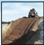
A trench excavated across the Hyden Fault scarp in south-west Western Australia showed that the scarp was formed by one or two large, shallow earthquakes of at least 6.0 magnitude.
