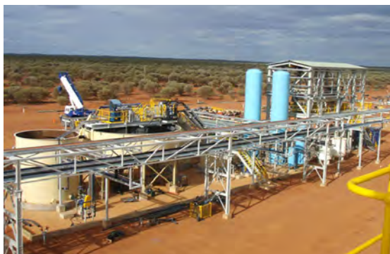
Figure 1.13. Filer press and thickener area at concentration plant, Mount Weld Project, Western Australia. Photographs provided by Georgia Bunn (Lynas Corporation Limited: http://www.lynascorp.com/ )
