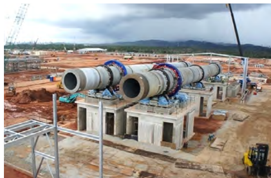
Figure 1.14. Installation of rotary kilns, Mount Weld Project, Malaysia. Photographs provided by Georgia Bunn (Lynas Corporation Limited: http://www.lynascorp.com/ )
