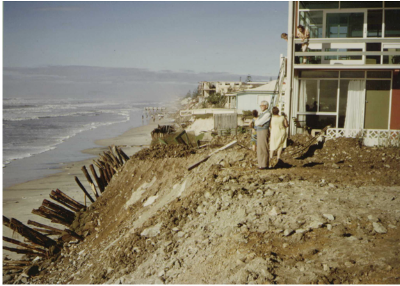
Figure 1. Severe beach erosion at Palm Beach during severe storms in 1967 (courtesy of EPA).
