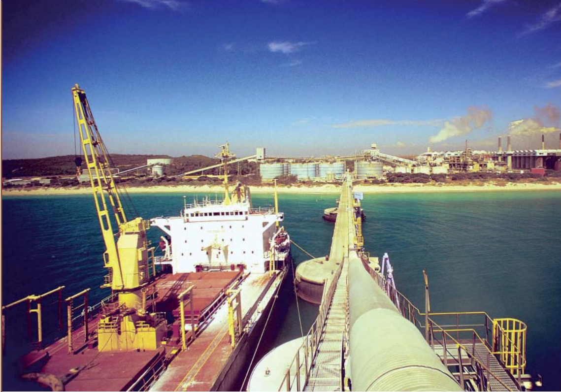
Bulk alumina loading facility in Kwinana, Western Australia (Alumina Ltd).
