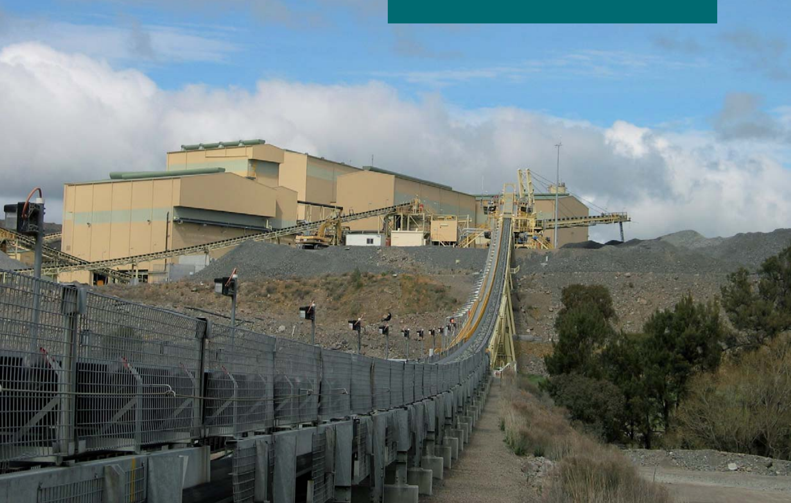
Ore conveyor from the underground Ridgeway gold-copper mine to treatment plant, New South Wales (Bill McKay, Geoscience Australia).
