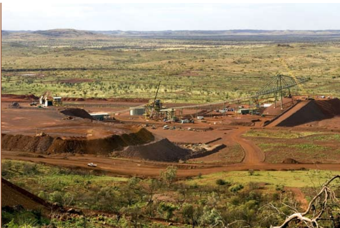
Infrastructure at the Orebody 18 mine, Western Australia (BHP Billiton Iron Ore Pty Ltd).
