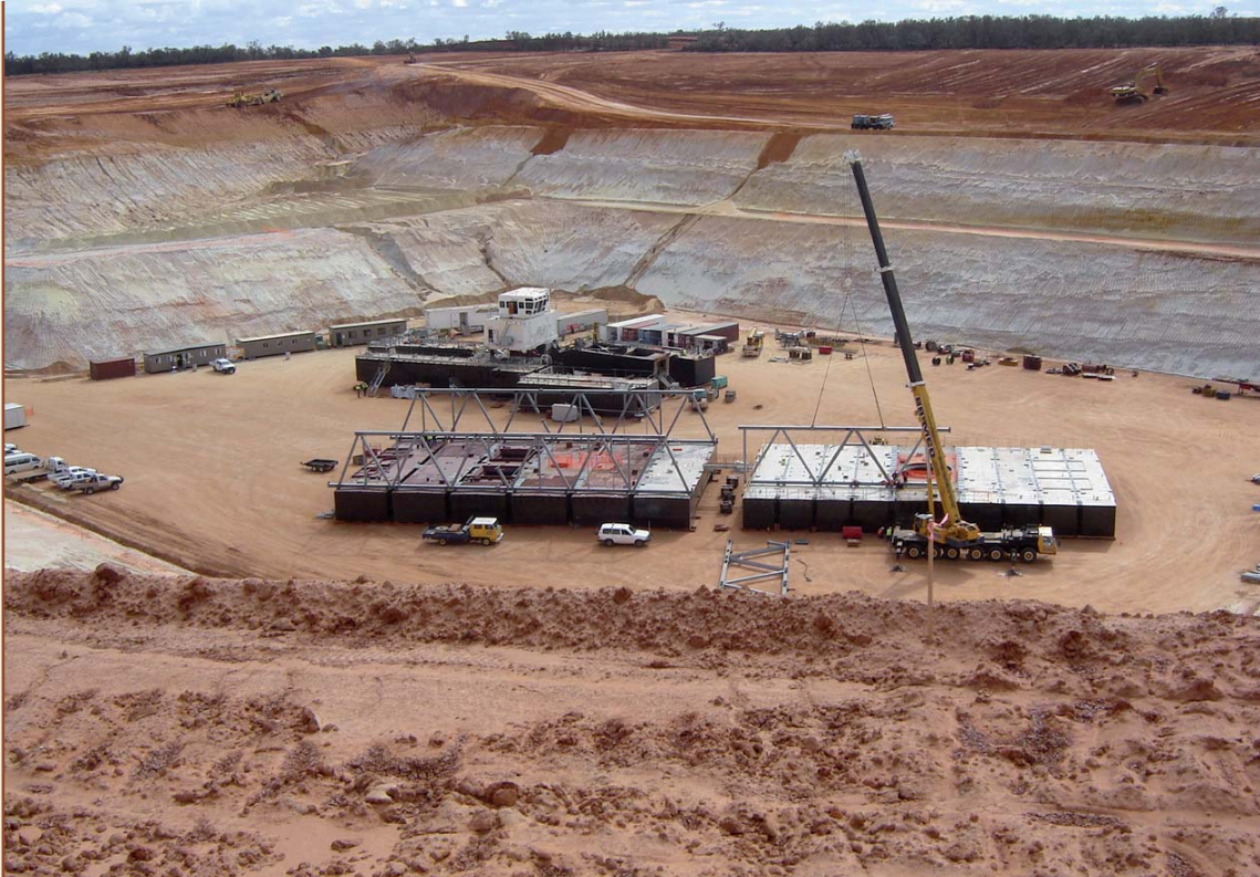
The Ginkgo Mine at the Pooncarrie Project showing Amanda II dredge and the floating concentrator being assembled in the bottom of the construction pit, New South Wales (Bemax Resources NL).
