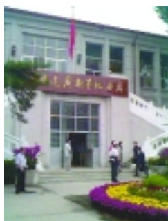
Main entrance to the China Remote Sensing Satellite Ground Station
