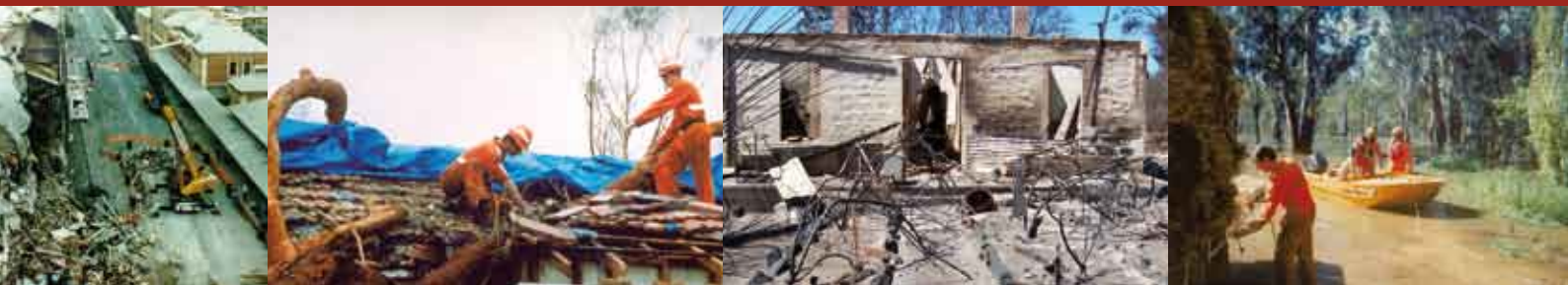
Building damage following an earthquake in Newcastle, New South Wales, December 1989 Photo courtesy: Geoscience Australia.
