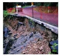
This landslide, on Lake Morris Road near Cairns, was triggered by heavy rain in March 1999.
